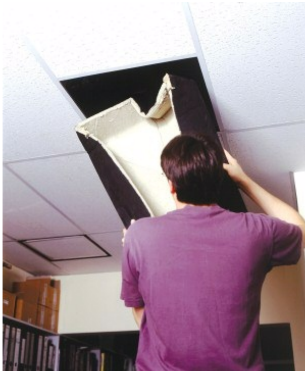
Installing luminaire cover
