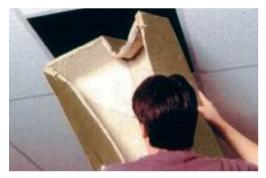
The Luminaire cover has been developed to provide maximum protection for ceilings where fire resistant tiles have been replaced by light fittings.
